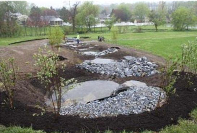
The RSC System is an open-channel conveyance structure that encourages surface flow to transition to shallow groundwater flow through a series of step-pools and riffles and an underlying sand/mulch bed. Can be adapted for moderately steep slopes.
