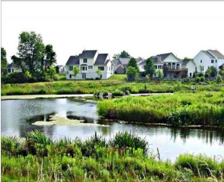
Wet ponds have a permanent pool of water and a landscaped fringe. Runoff from each storm enters the pond and raises the normal water level, and the outlet structure releases the runoff at a slower rate. This “draw down” or holding time allows pollutants to settle to the bottom while also reducing the discharge.
