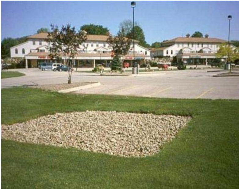
Infiltration practices utilize temporary surface or underground storage to allow incoming stormwater runoff to infiltrate into underlying soils. Runoff first passes through multiple pretreatment mechanisms to trap sediment and organic matter before it reaches the practice.
