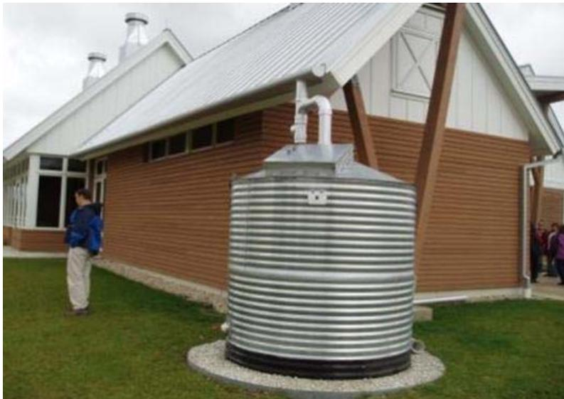
Rainwater Harvesting systems provide for the capture, storage, and release of rainwater for future beneficial use, either inside or outside the building. Systems usually capture rooftop runoff. Storage tanks can be a variety of materials and either above ground or underground.
