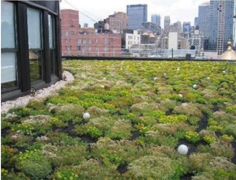
Vegetated Roofs are an alternative roof surface that typically consists of waterproofing and drainage materials and an engineered growing media that is designed to support plant growth.
