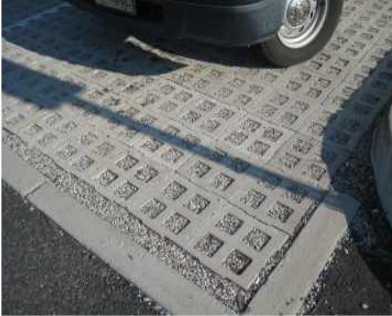
Permeable Paving materials include concrete, asphalt, and interlocking pavers that allow runoff to filter through voids into a gravel storage reservoir.
