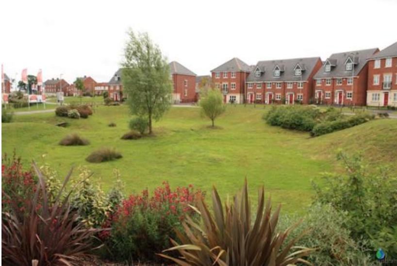
Dry (Extended Detention) Ponds do not have a permanent pool, and remain dry except during and shortly after storm events. Some extended detention facilities may have a wet marsh with plantings in the bottom for additional pollutant removal.
